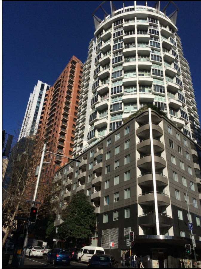
Figure 8: View of the mixed-use development at 298-304 Sussex Street (known as Maestri Towers), on the southern side of Bathurst Street
