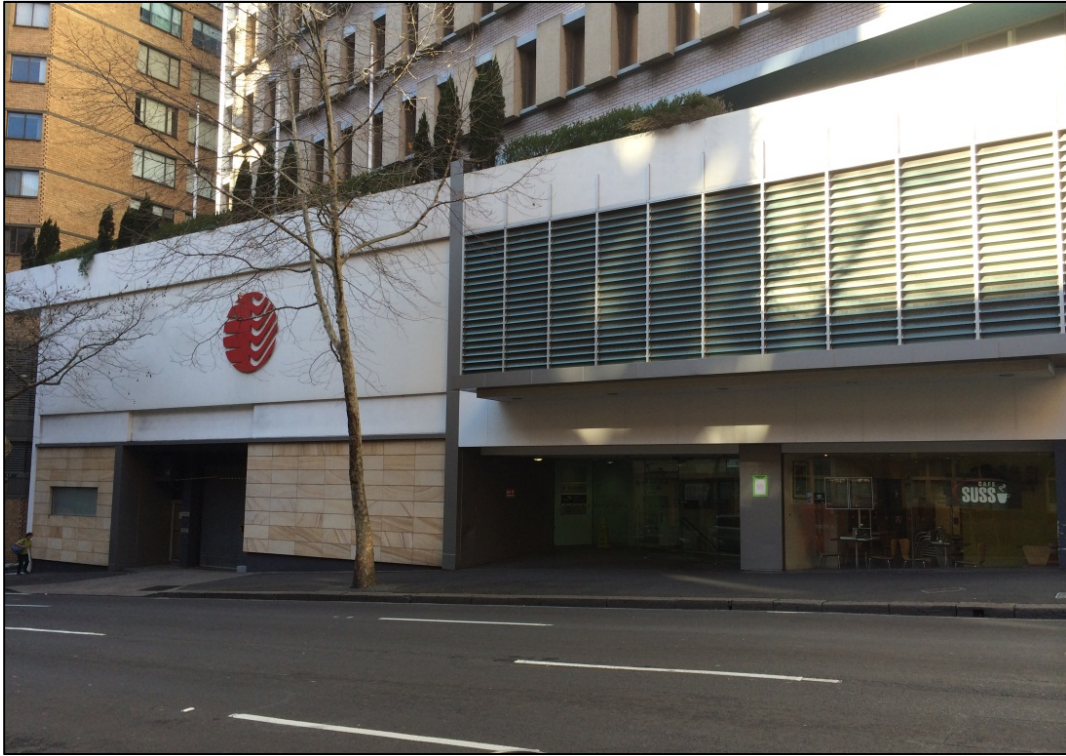
Figure 4: The existing ground floor retail and vehicular access to the site on its Sussex Street frontage
