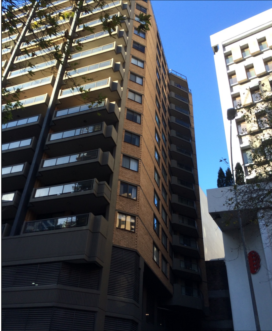
Figure 18: View of the southern elevation of the Newhaven residential building
